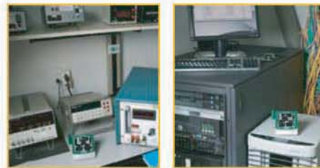
Monitoring humidity and temperature levels in a calibration laboratory or server room
